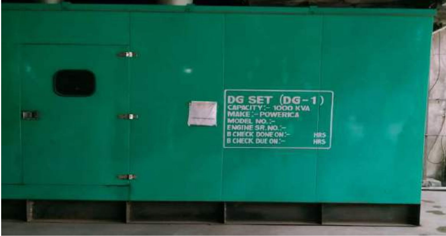
DG Acoustic Enclosure 1000KVA
