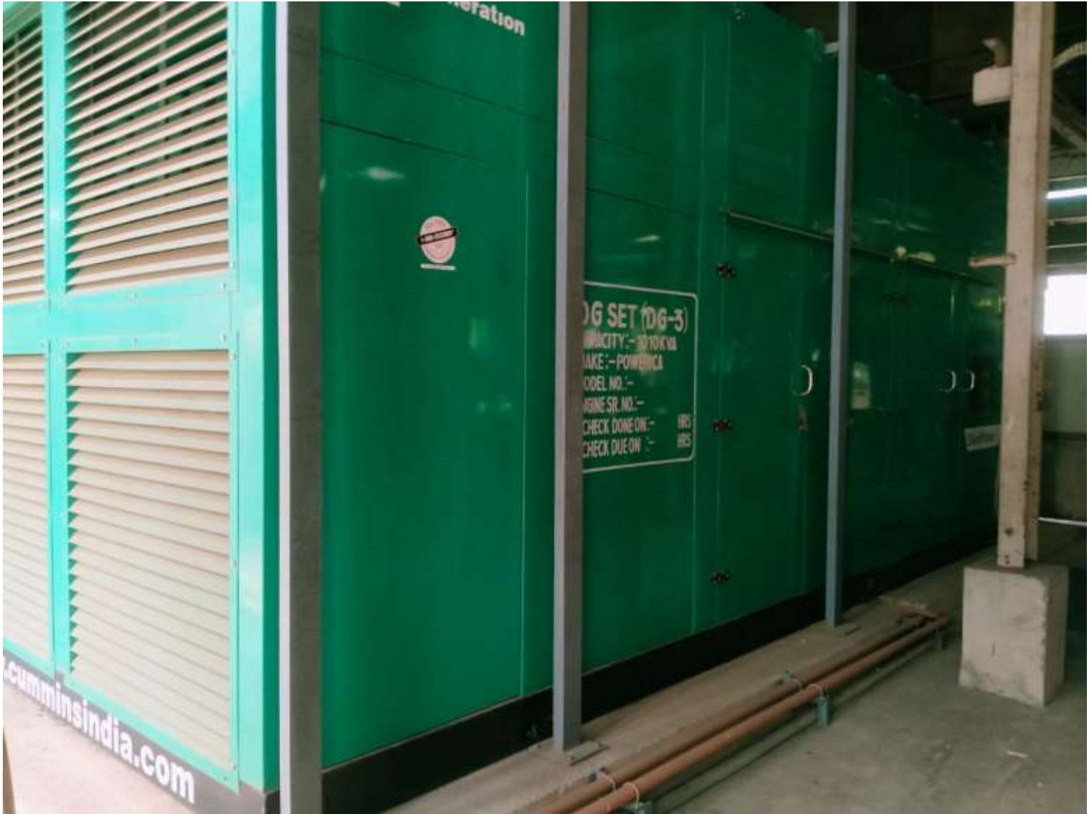
DG acoustic Enclosure for 1010 KVA
